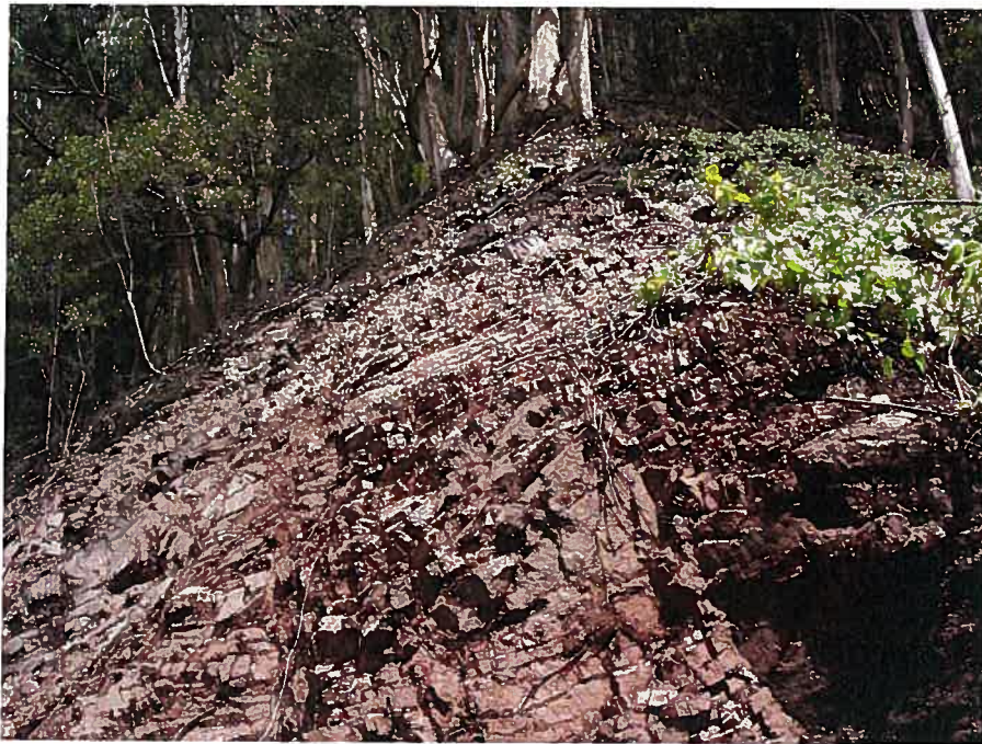
Picture #7: Unstable hillside that falls into yards below.
