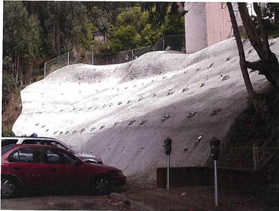
Picture #12: Concrete abutment with rock bolts at base of Kirkham Apartments
